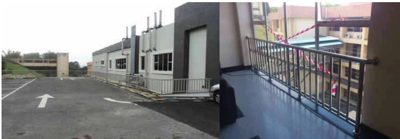
Foto 12.2: Rail keselamatan kawasan bangunan PTK Photo 12.2: Safety railing of PTK Building
