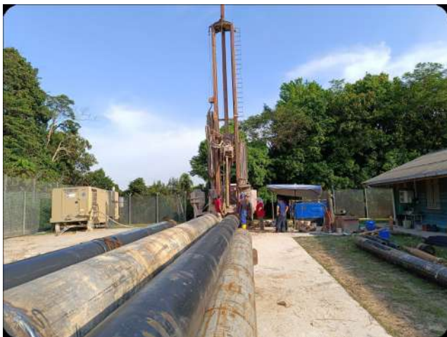
Figure 3: Borehole construction using Foremost Dual Rotary DR 24 mounted drilling rig truck.
