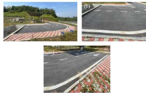
Figure 1: (a) Evaluation Verification Facility (EVF) (b) 1 st phase scanning area (c) 2 nd phase scanning area
